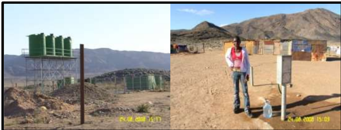
Figure 46. Illustration of water supply infrastructure in Tutangeni informal settlement in Rosh Pinah, Namibia (2008).
