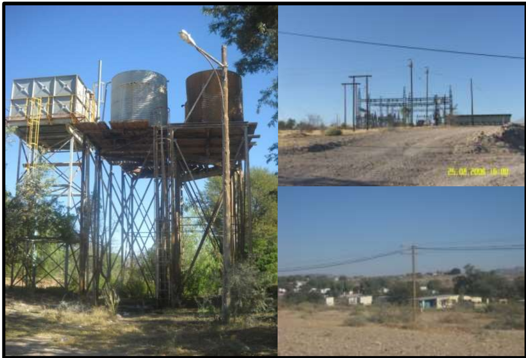
Figure 73. Illustration of municipal infrastructure in Klein Aub, Namibia (2010).
