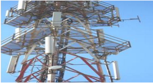
Figure F1: Telecom LTE panels on an eNodeB, Walvis Bay
