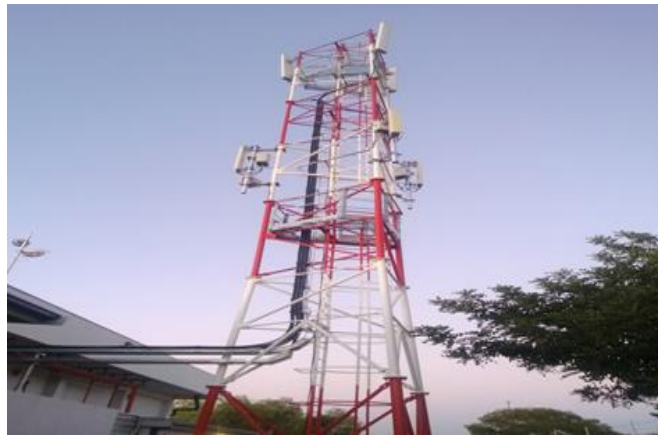
Figure 5.4 LTE base station
