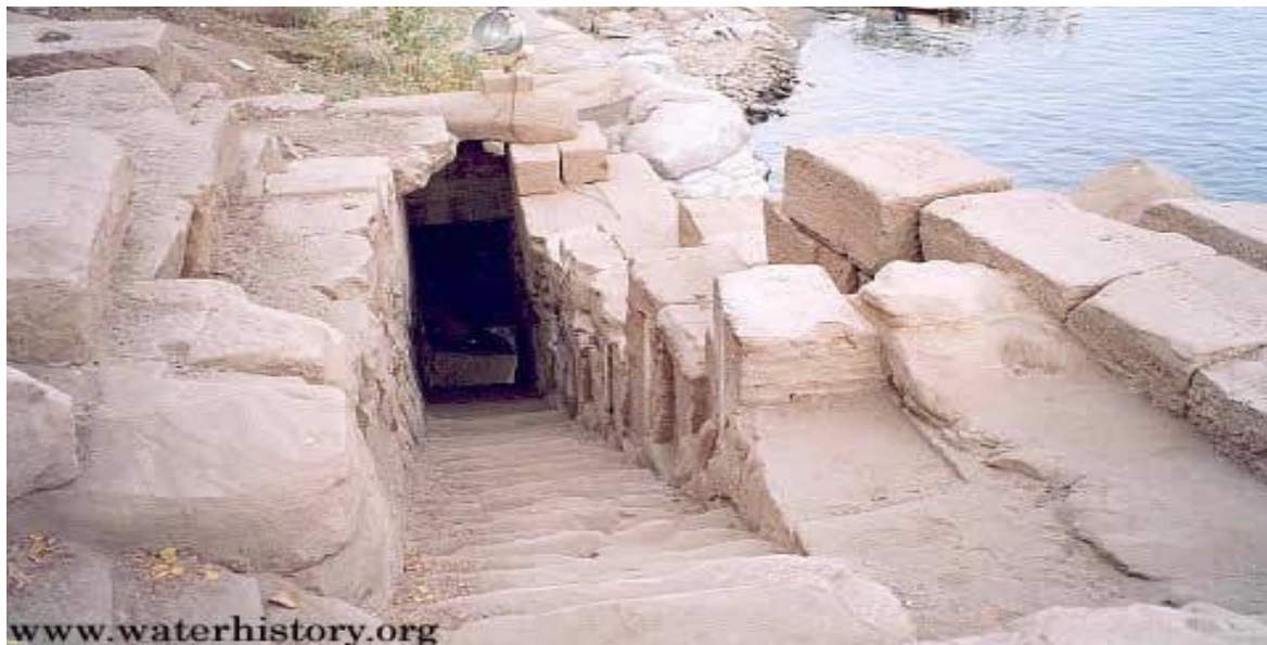
Figure 2.4 : The nilometer on Elephantine Island, Aswan, consists of stairs and staff gauges.
