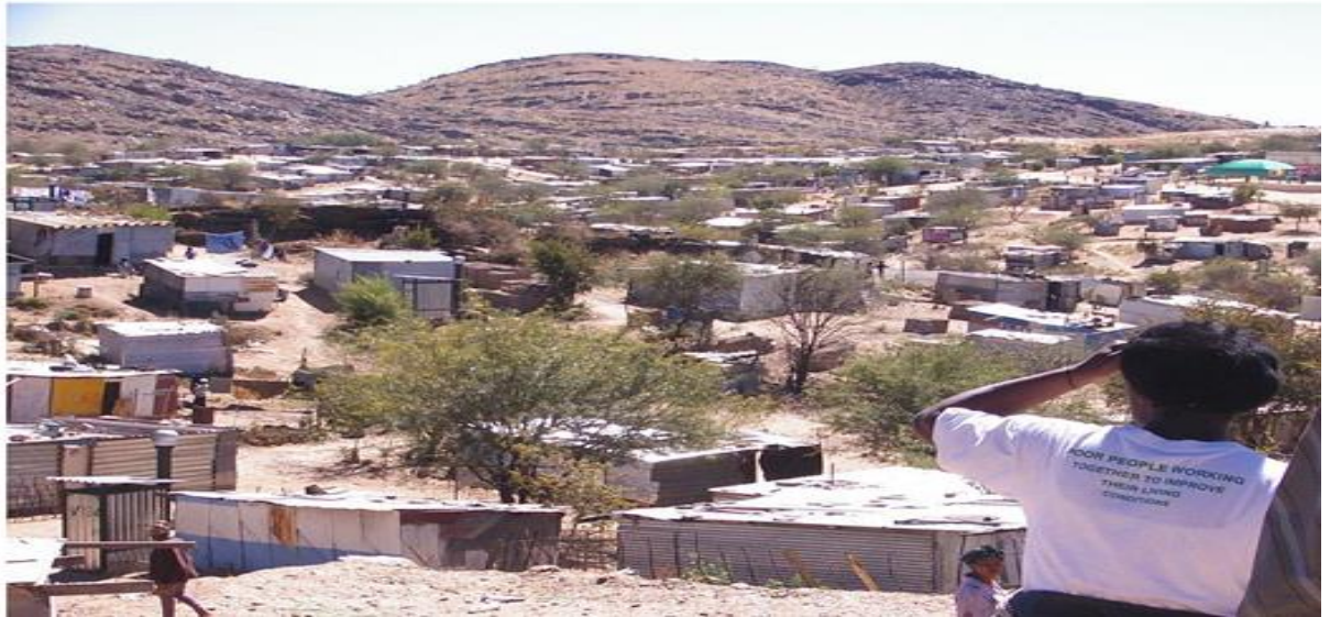
Figure 3.2 Havana Informal Settlement
