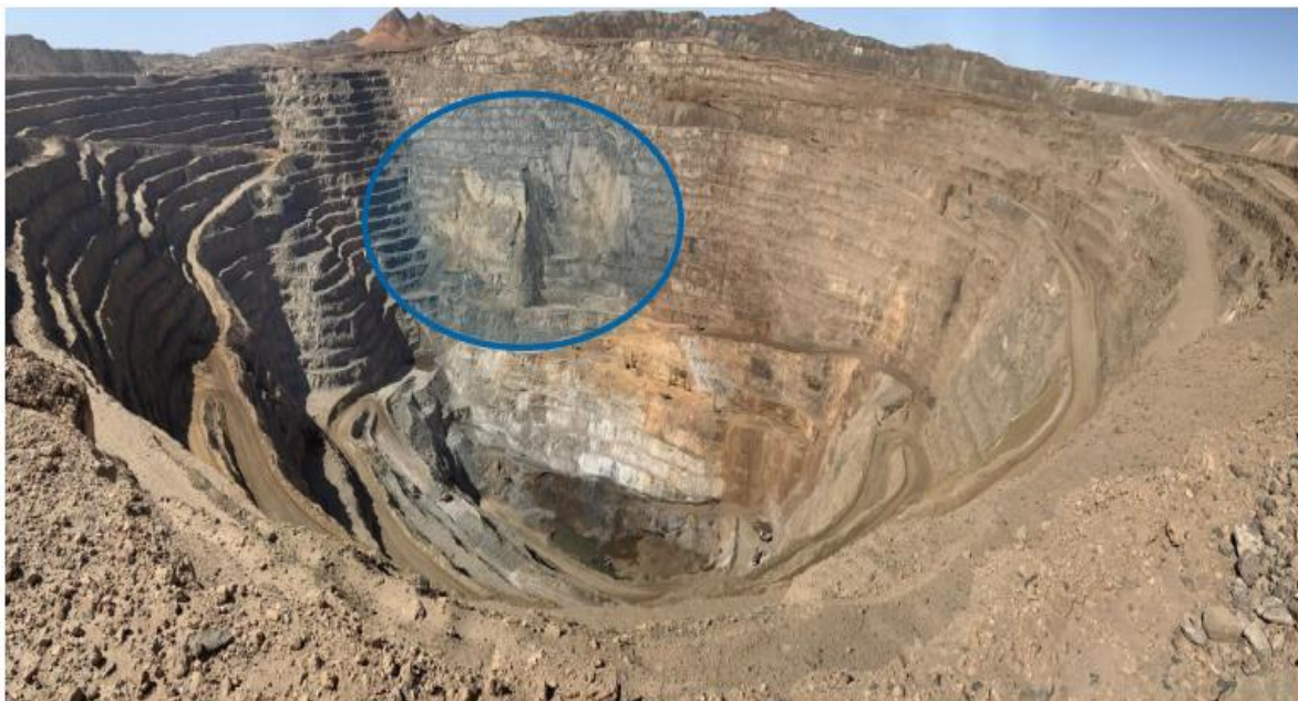
Figure 72: The slope failure spot at Skorpion Zinc Mine
