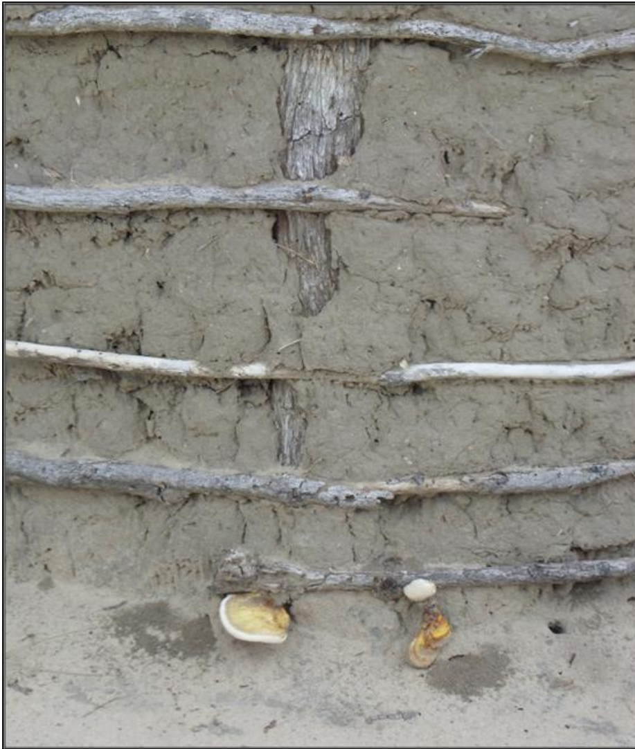
Appendix 1d. Ganoderma isolates on building posts
