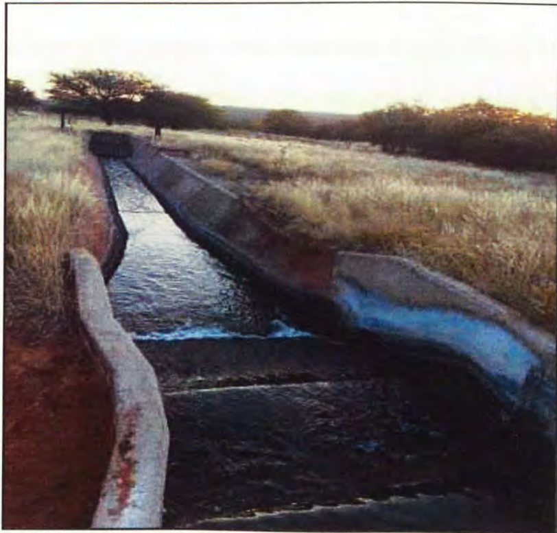
Figure 3-2 Open canal section at flume 3
