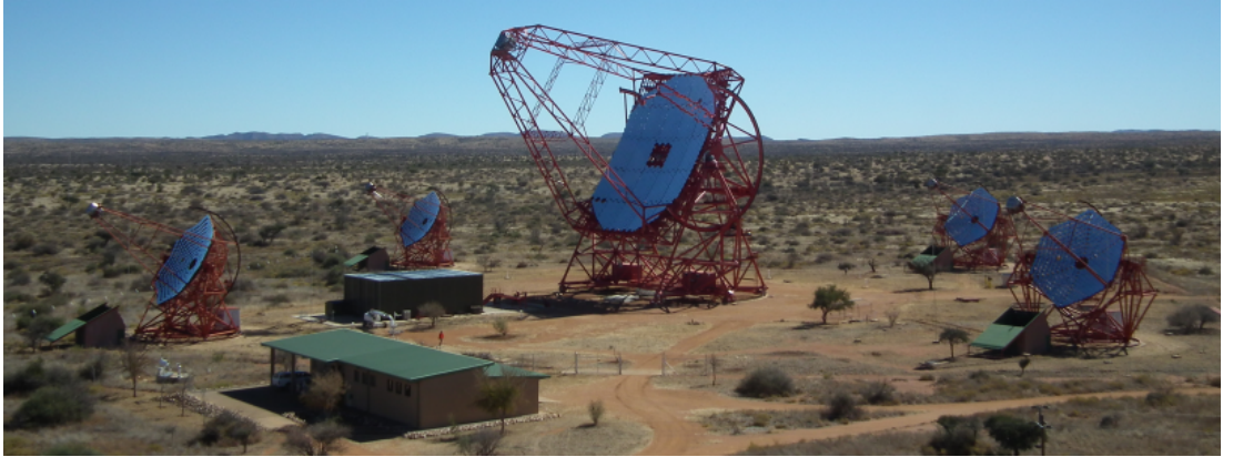
Figure 3.1. The H.E.S.S. telescope system in the Khomas highland of Namibia, located at an elevation of 1.8 km above sea level. H.E.S.S.-I is arranged in a square of 120 m sides operating in stereoscopic mode, with CT5 at the center of the array [1]. This setup was chosen because the typical radius of the cone of Cherenkov light is \approx 120 m. Also, this setup allows for multiple telescopes to observe the same Cherenkov event, allowing the use of stereoscopy.
