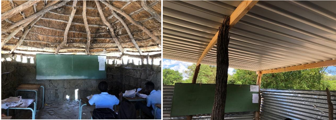
Figure 1. Two classrooms at School B
