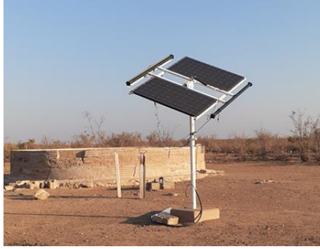
Figure 3.8. Solar powered borehole at Laurencia.
