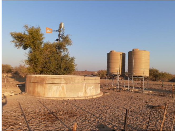
Figure 3.12. Cement dam and water tanks at Laurencia Pos
