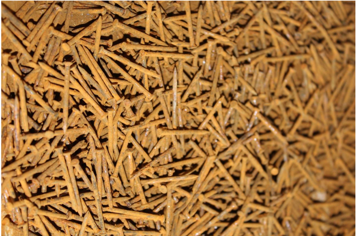
Figure 6 - Nails covered with bright orange rust. Photograph: By Author
