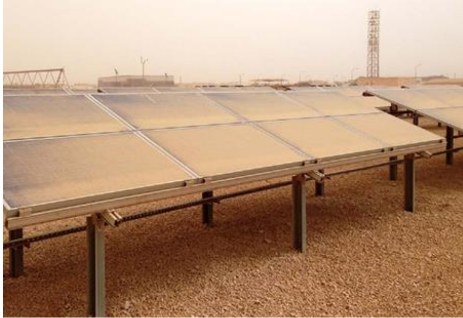
Figure 2.1. Illustration of soiling on solar cell cover glass
