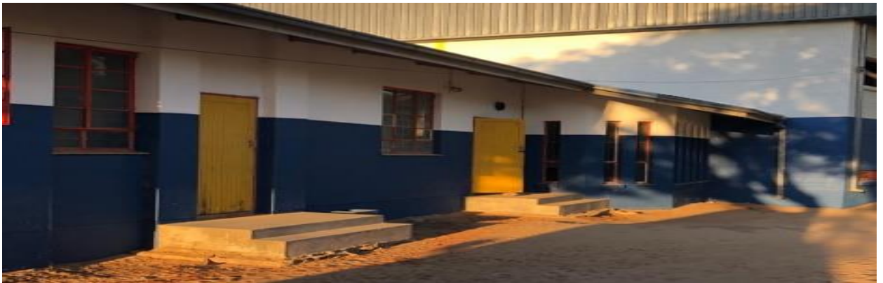
Figure 4.4 School B: Pavements and Stairs to the Learning Areas
