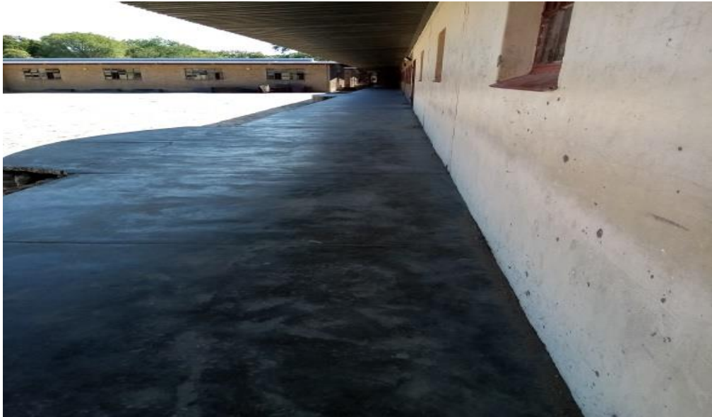
Figure 3.2 Facilities at School A: Hostel and Dining Hall Side View
