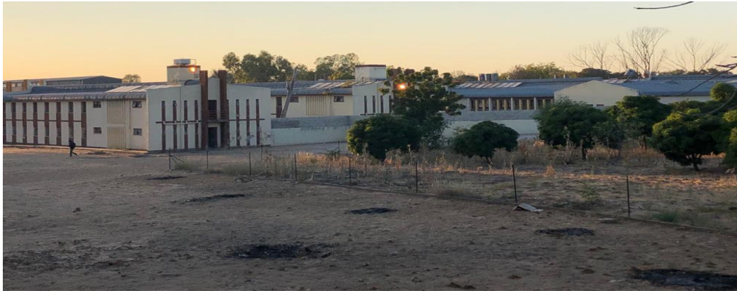
Figure 3.4 Overview of School B: School Hostel Side
