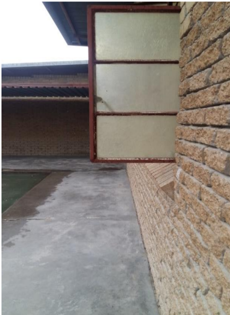
Figure 4.6 School A: Protruding Window and Wall with Rough Bricks
