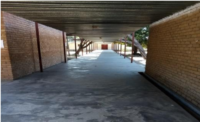
Figure 4.3 Pavement with Metal Poles Learners Have to Jump to Go to the Garden and Sports Field
