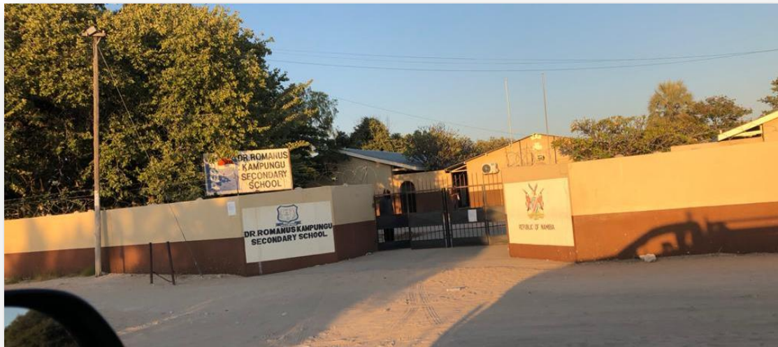
Figure 3.3 Entrance of School B
