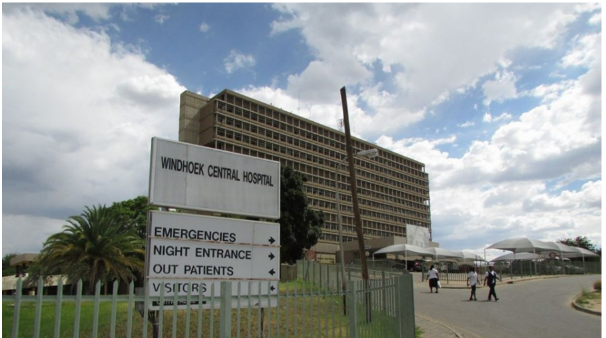
Figure 1: Windhoek Central Hospital
