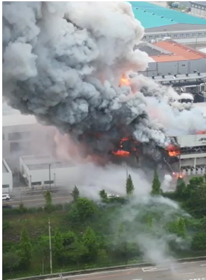
Figure 16. The BESS fire eruption in Hwaseong, Gyeonggi Province [47].
