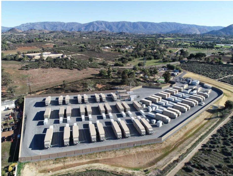
Figure 9. Southern California’s Valley Centre Energy Storage Project [39].
