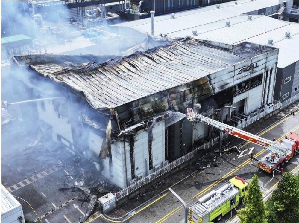
Figure 17. Hwaseong, South Korea, battery fire aftermath [47].
