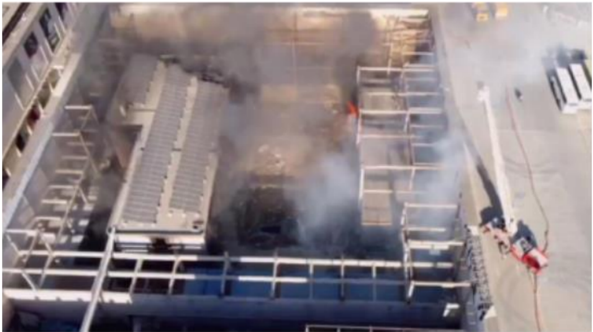
Figure 12. The power station after the fire accident [12].
