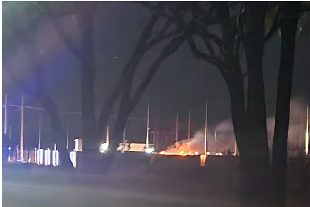
Figure 7. The Australia, Queensland, Bouldercombe fire incident [38].
