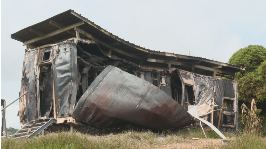
Figure 13. Saint-Esprit, Martinique, France, fire and explosion accident [44].
