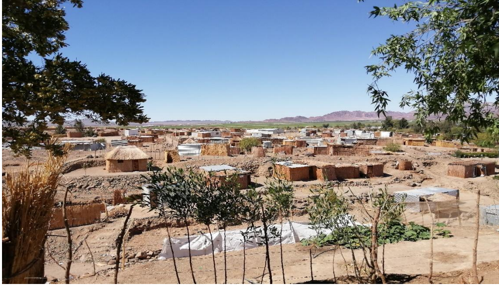
Figure 4 The type of housing structures in the settlement- Area 5 (Source: Tjitombo, 2020).
