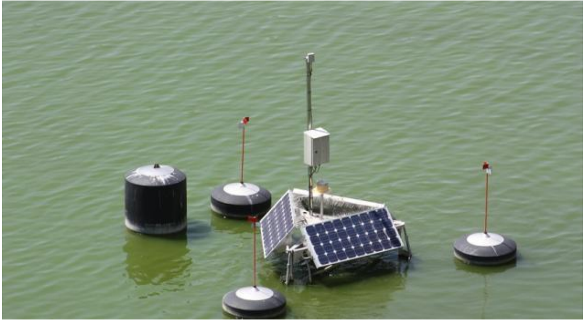
Figure 6: Solar bees floating on Swakkoppoort dam, Namibia (Meding, 2016).
