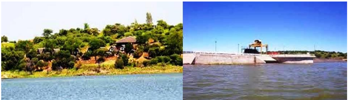
Figure 16: Von Bach dam (Tungenicom, 2016; Namwater, 2016).
