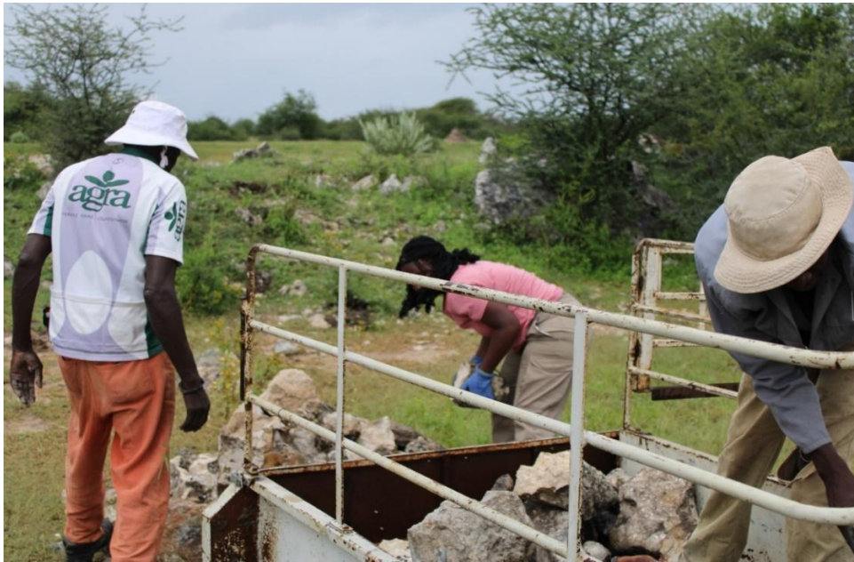
Figure 1: Community members collecting stones to build a mushroom house
