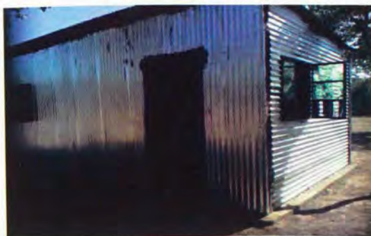
Figure 4.7(a): Exterior of a pre-primary classroom (mobile school X)
