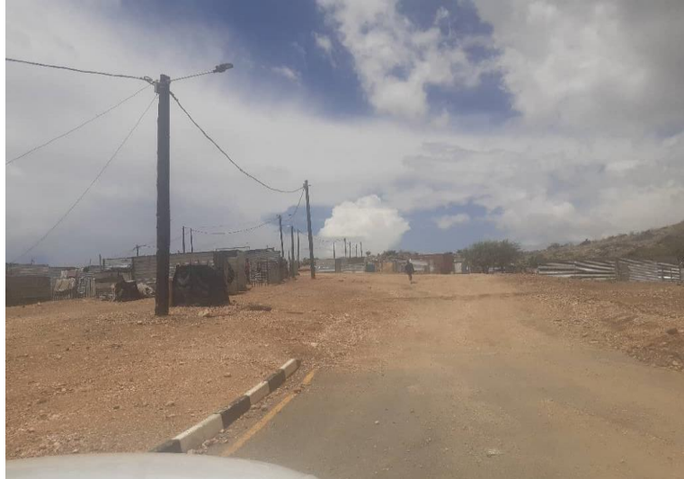
Figure 4.31: Electrification of 1000 households in Tobias Hainyeko Constituency
