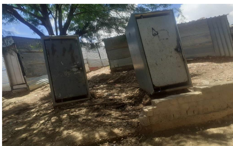
Figure 4.34: A shared ablution facility in Kilimanjaro location, Tobias Hainyeko Constituency
