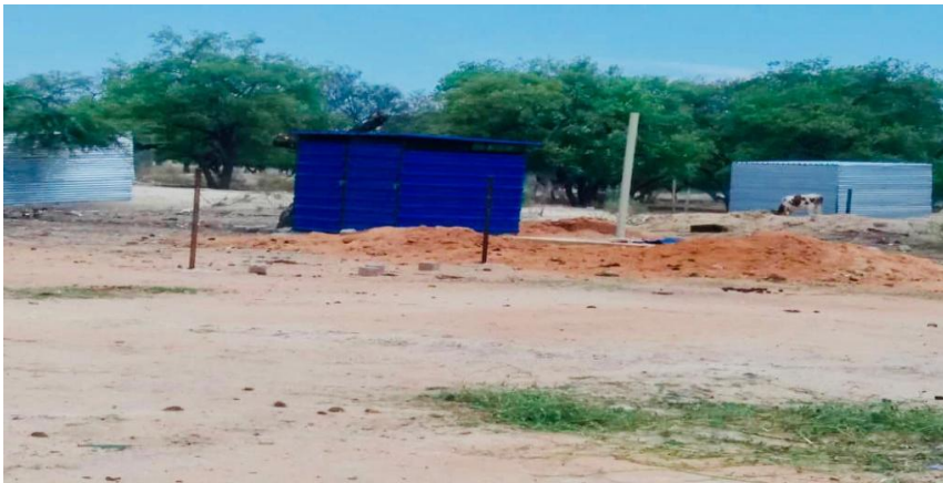
Picture 2.4 Septic tank used by residents of Okalongo Settlement.
