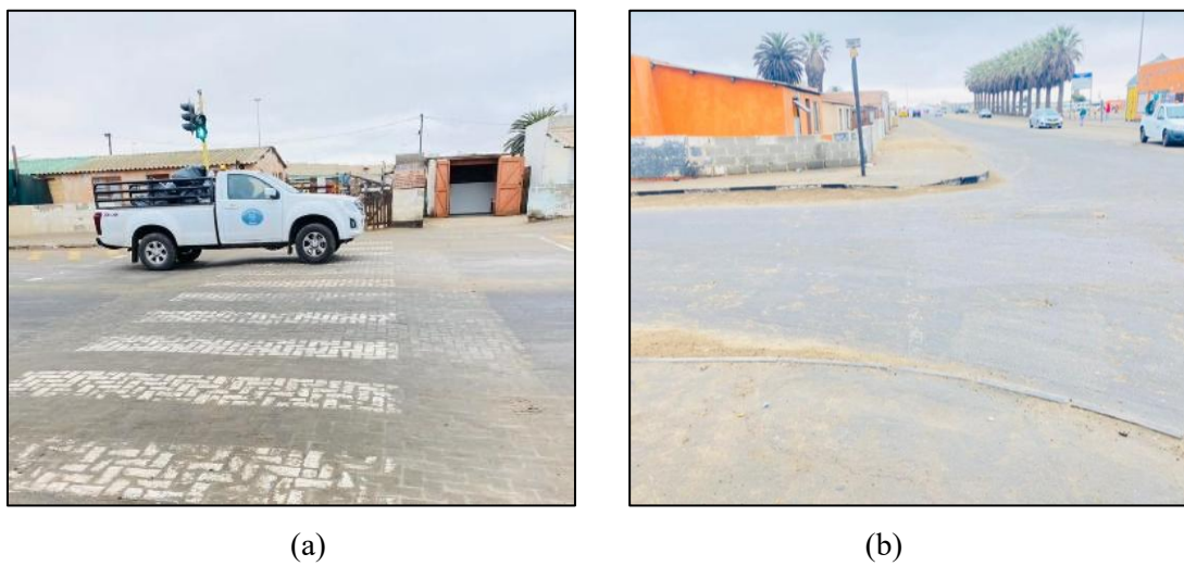
Figure 5.27: (a) Drivers ignoring traffic signals at pedestrian crossings; (b) Poor crosswalk visibility
