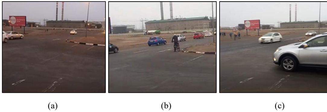
Figure 5.19: (a) Poor crosswalk visibility; (b) Lack of crosswalks on pedestrian-desired crossing lines; (c) Drivers failing to yield at pedestrian crosswalks
