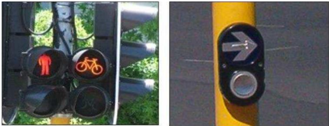
Figure 2.6: Pedestrian and cyclist audible and vibro-tactile traffic signal, adopted from (SANRAL and ITS, 2017)
