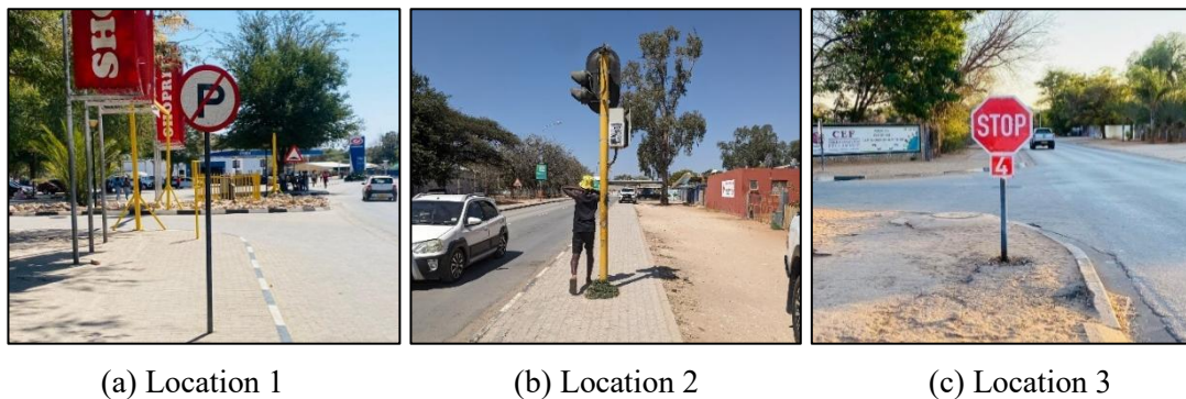
Figure 5.7: Obstructions (poles) along sidewalks
