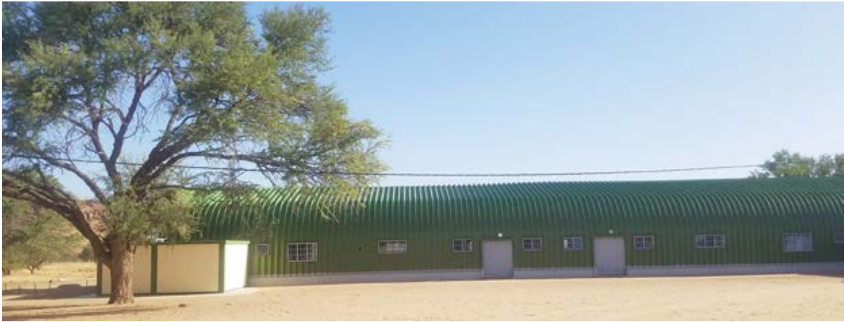
Figure 71: An earthquake-resistant hostel block constructed recently in Anker for Edward //Garoeb Primary School, Kunene Region
