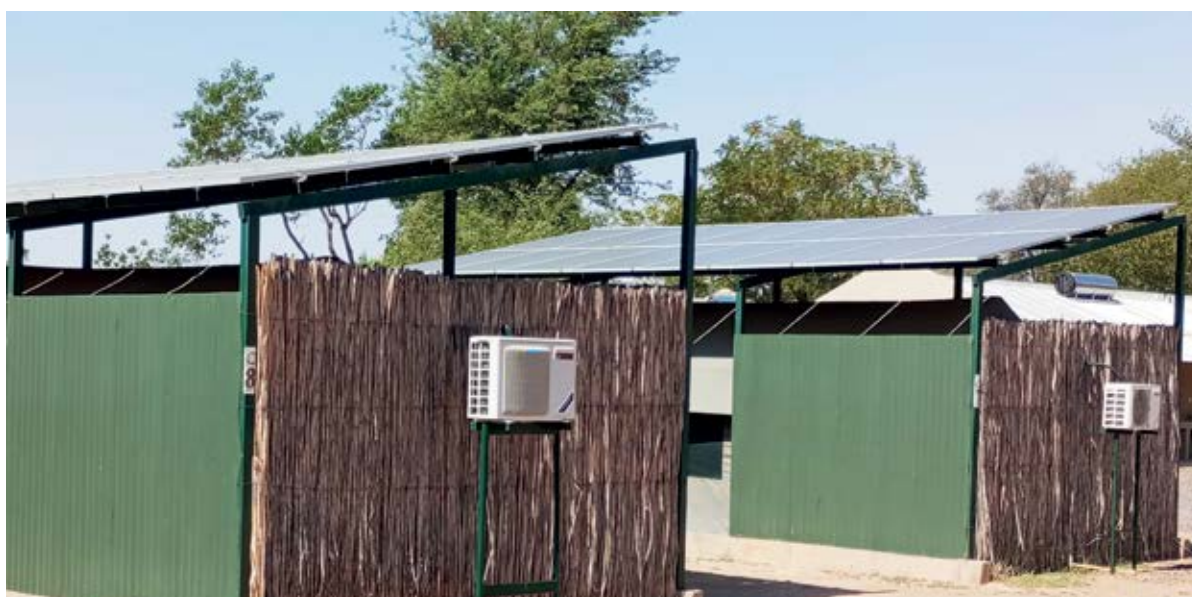
Figure 46: An example of the air condition system powered by solar panels on a partially thatched structure in southern Namibia
