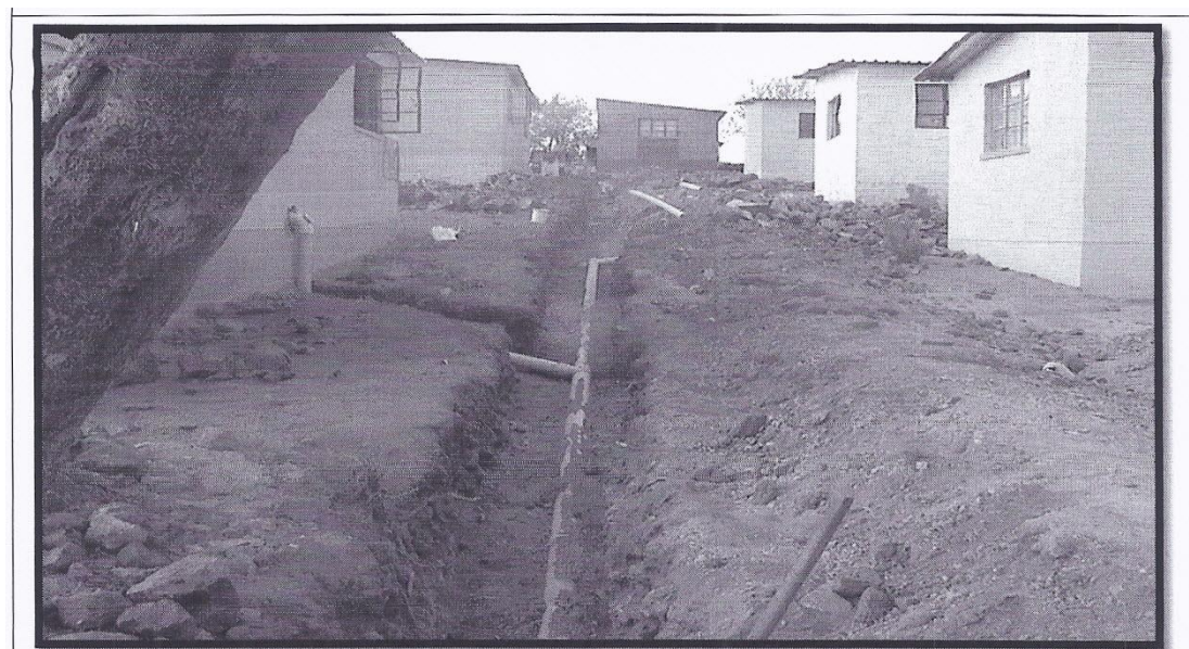
Photo 1.1: Okahandja Park: Excavated trench and fitted sewerage pipes by community and upgraded houses
