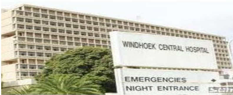
Figure: 3.1: Windhoek Central Hospital (Source: (Ngatjiheue, 2020))
