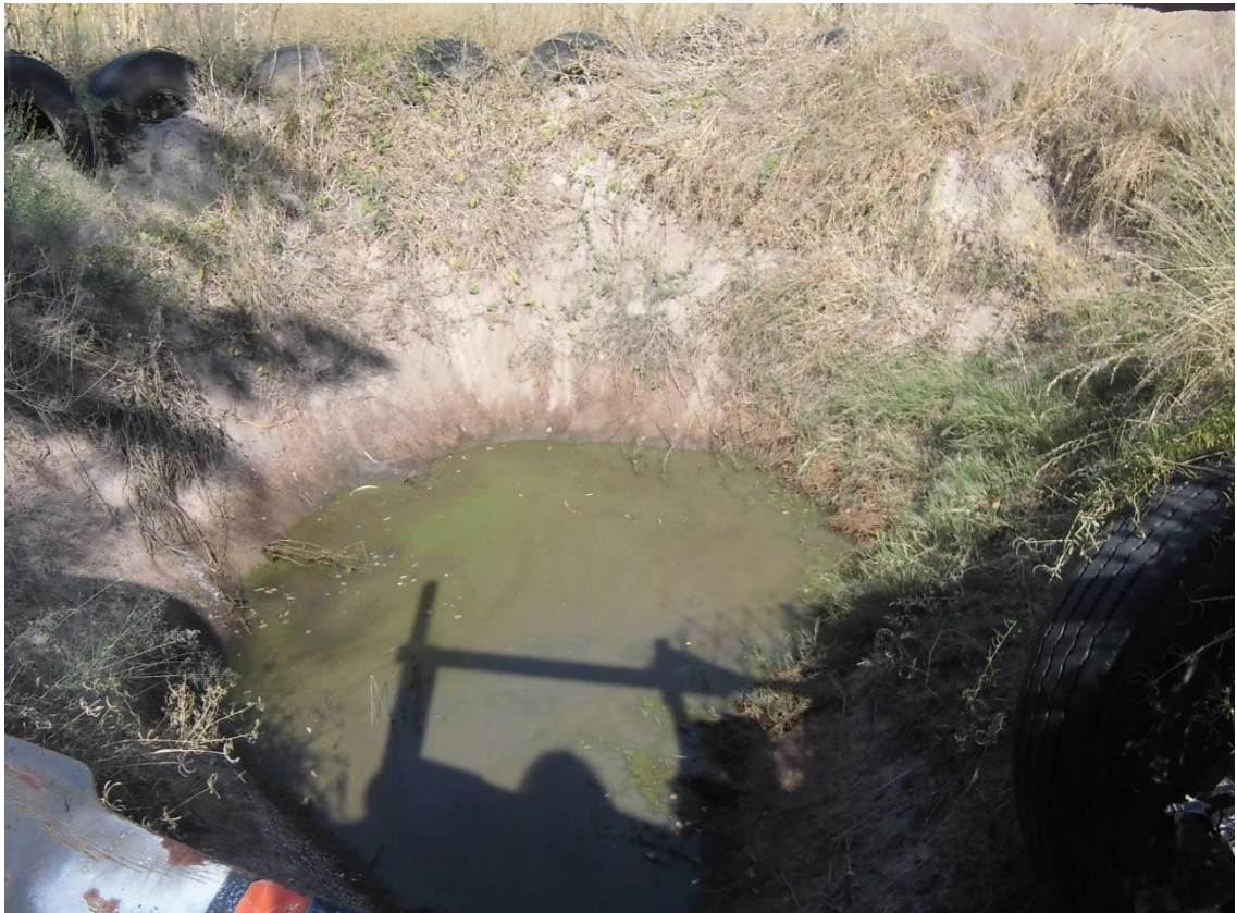
Figure14: Dug well at Oshikango informal settlement
