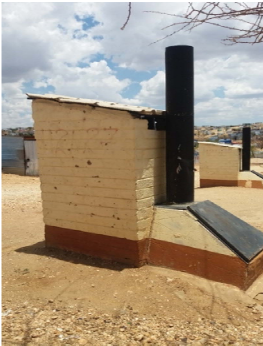
Pictures 8 and 9: The individual Otji toilet with a regular toilet seat
