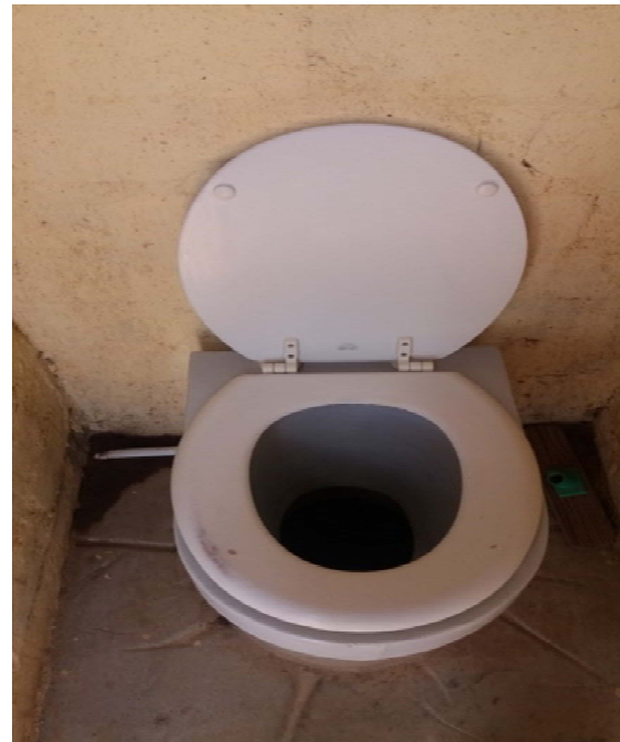
Pictures 8 and 9: The individual Otji toilet with a regular toilet seat
