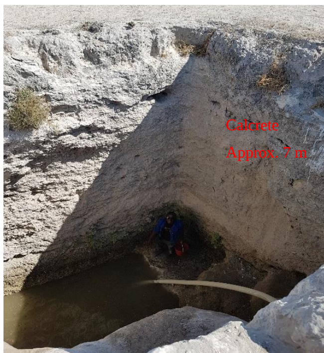
Figure 4-5: Examples of hand-dug wells in Omusati region
