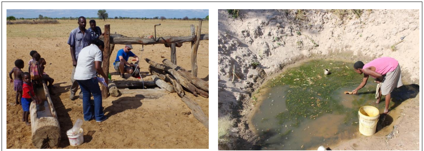
Figure 4-4: Two types of hand-dug wells: a) the deep wells (cylindrical-shaped hand-dug wells) known as “Eendungu” and b) shallow wells (funnel-shaped hand-dug wells) locally known as “Omifima”
