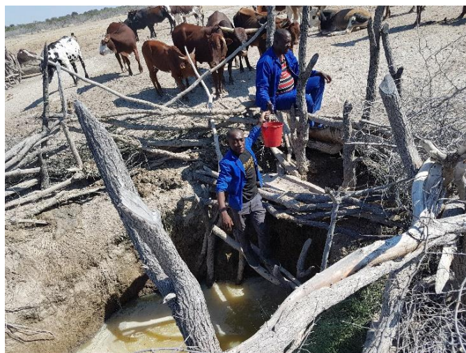
Figure 4-5: Examples of hand-dug wells in Omusati region
