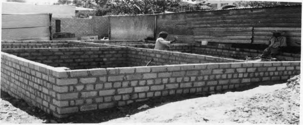
Photo 5: House underconstruction: Hakahana area
