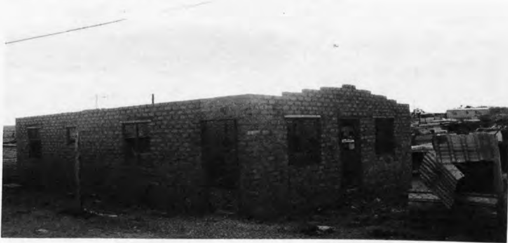
Photo 3: Incomplete spacious house: Goreangab area
