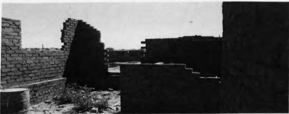
Photo 6: Incomplete big house: Khomasdal area
