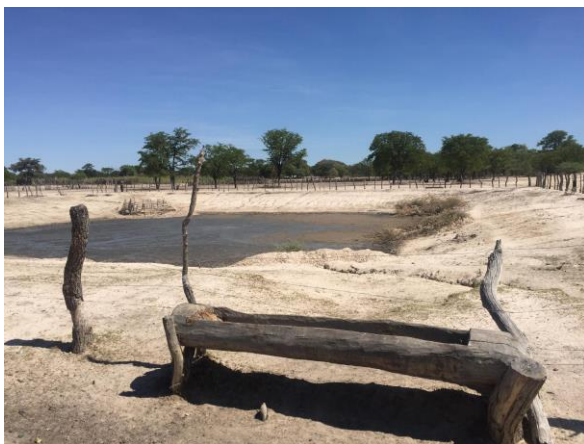
Figure 4.10 (a) Ekangolangobe earth dam
