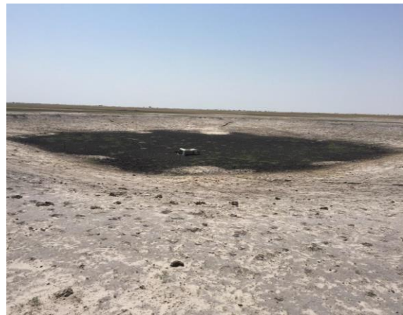
Figure 4.6 Sigopi earth dam silting up
