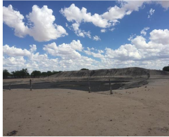
Figure 4.8 Enongo earth dam
