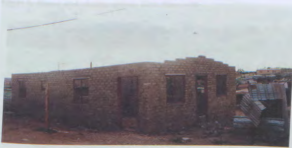
Photo 3: Incomplete spacious house: Goreangab area
