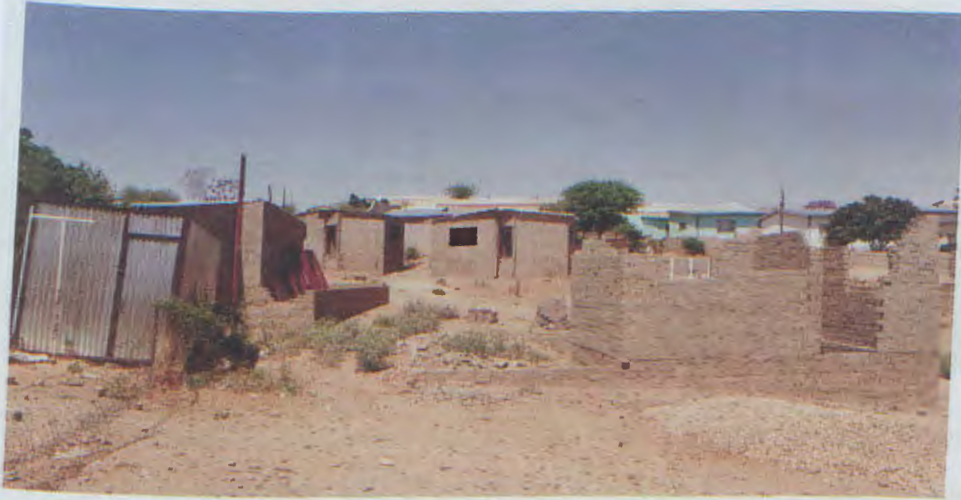
Photo 1: Incomplete houses: Khomasdal area
