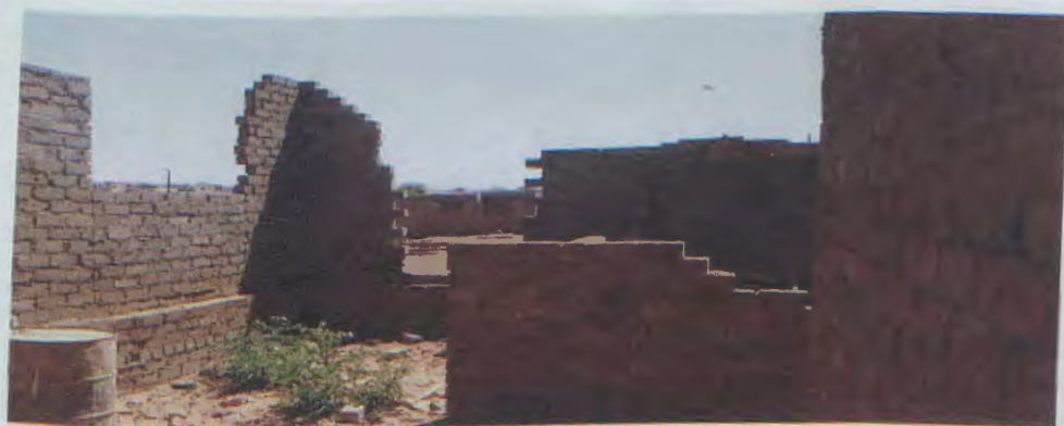
Photo 6: Incomplete big house: Khomasdal area
