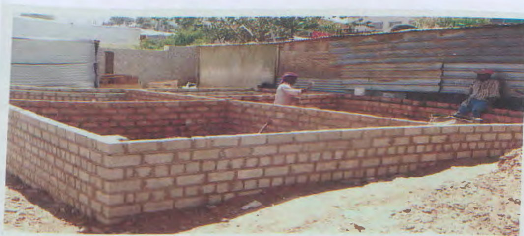
Photo 5: House underconstruction: Hakahana area
