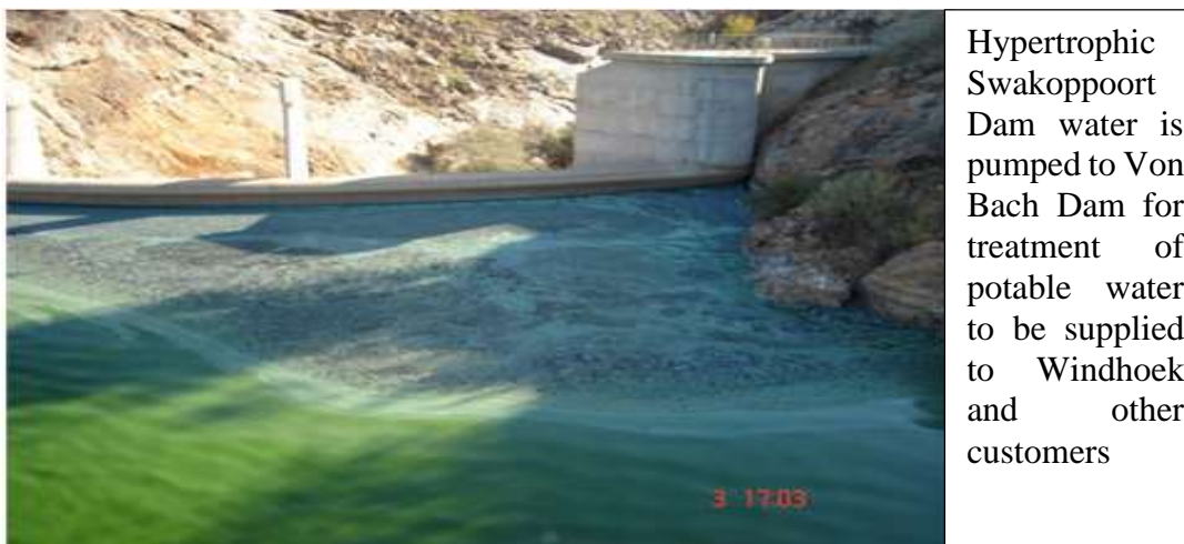
Figure 7.5 Swakoppoort Dam Algae Picture (2011)
