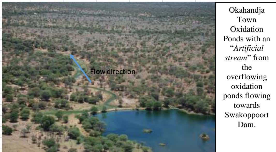
Figure 7.4 Okahandja Oxidation Pond Spilling Toward Swakoppoort Dam (2011)
