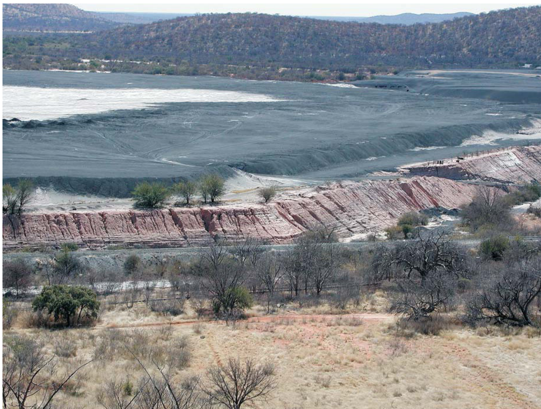
Figure 6.2: Part of the old tailings impoundment in the Tsumeb Smelter Area viewed from the south. Fine-grained tailings (pinkish brown) are partly covered by coarse-grained fractions of slag mill tailings (black) to suppress dust (Křibek & Kamona, 2005).
