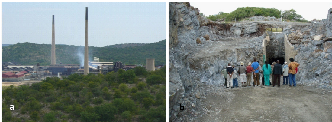
Figure 5.4: TCL infrastructural development: (a) the Tsumeb Smelter and (b) an adit at Kombat.
