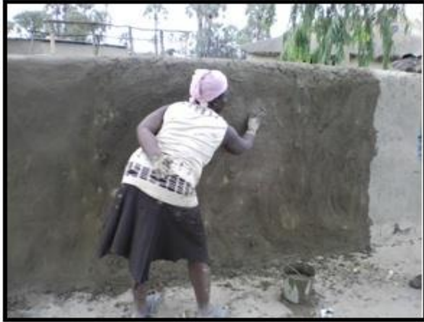
Figure 48: House fence renovation after the flood (September, 2011).
