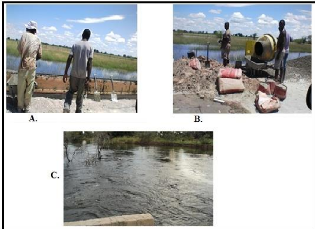
Figure 22: Gravel roads and small culverts under construction (March, 2011).
