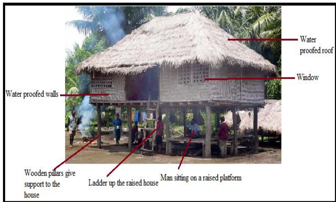
Figure 15: Raised house in Papua New Guinea [Source: Mercer, 2006].
