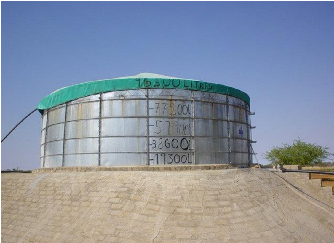
Figure 1.1: Main Water Tank
